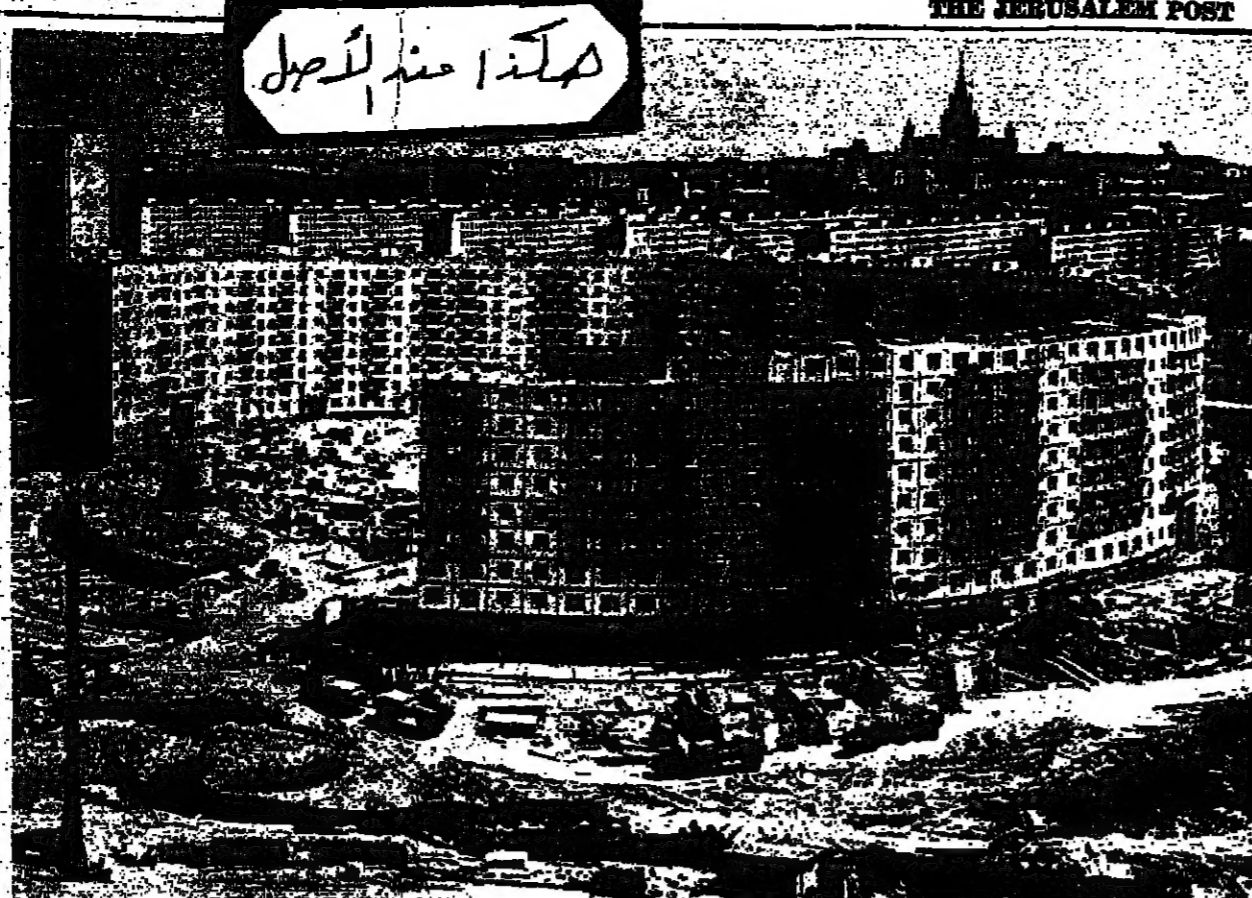
Moscovites will soon be living in the 800 flats that make up this nine-storey circular building, which includes playgrounds and leisure areas, now being built in the Soviet capital.
